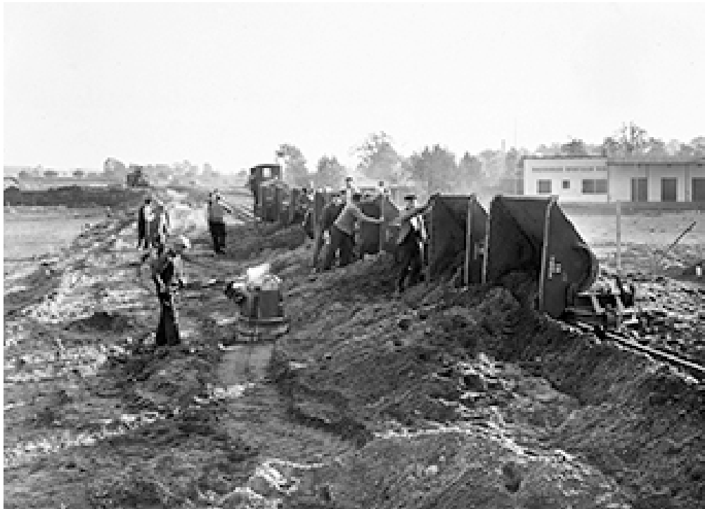
Fig. 2: Reichsautobahn under construction, in Radeburg (Saxony), 1937; a four-metre-high dam is built with manual labour (SLUB/Deutsche Fotothek, Walter Möbius)
